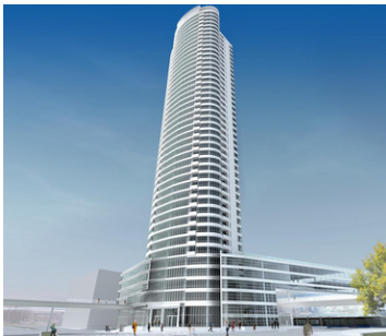
Countertop installation at the Couture in downtown Milwaukee will take place in summer 2023.
